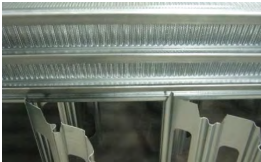
Images 4 and 5 – Positioning Heavy-Duty Perforated floor plank in SuperWave Supports
