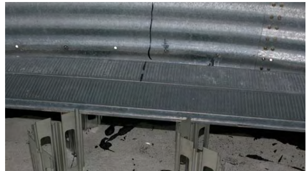
Image 3 – Marking bin wall, installing first plank
