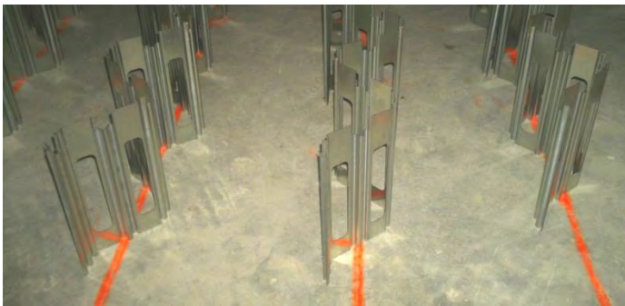
Image 2 – Positioning SuperWave Supports
