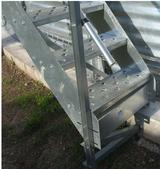
Image 4 – Connecting bottom stair to bin
