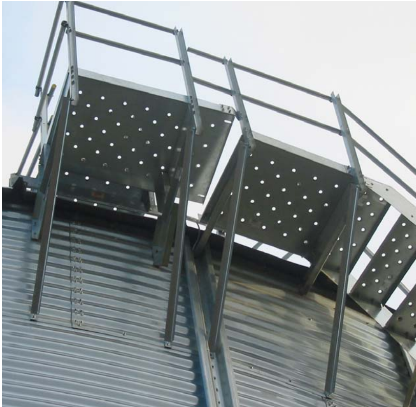
Image 2 – Roof stairs and manhole platforms
