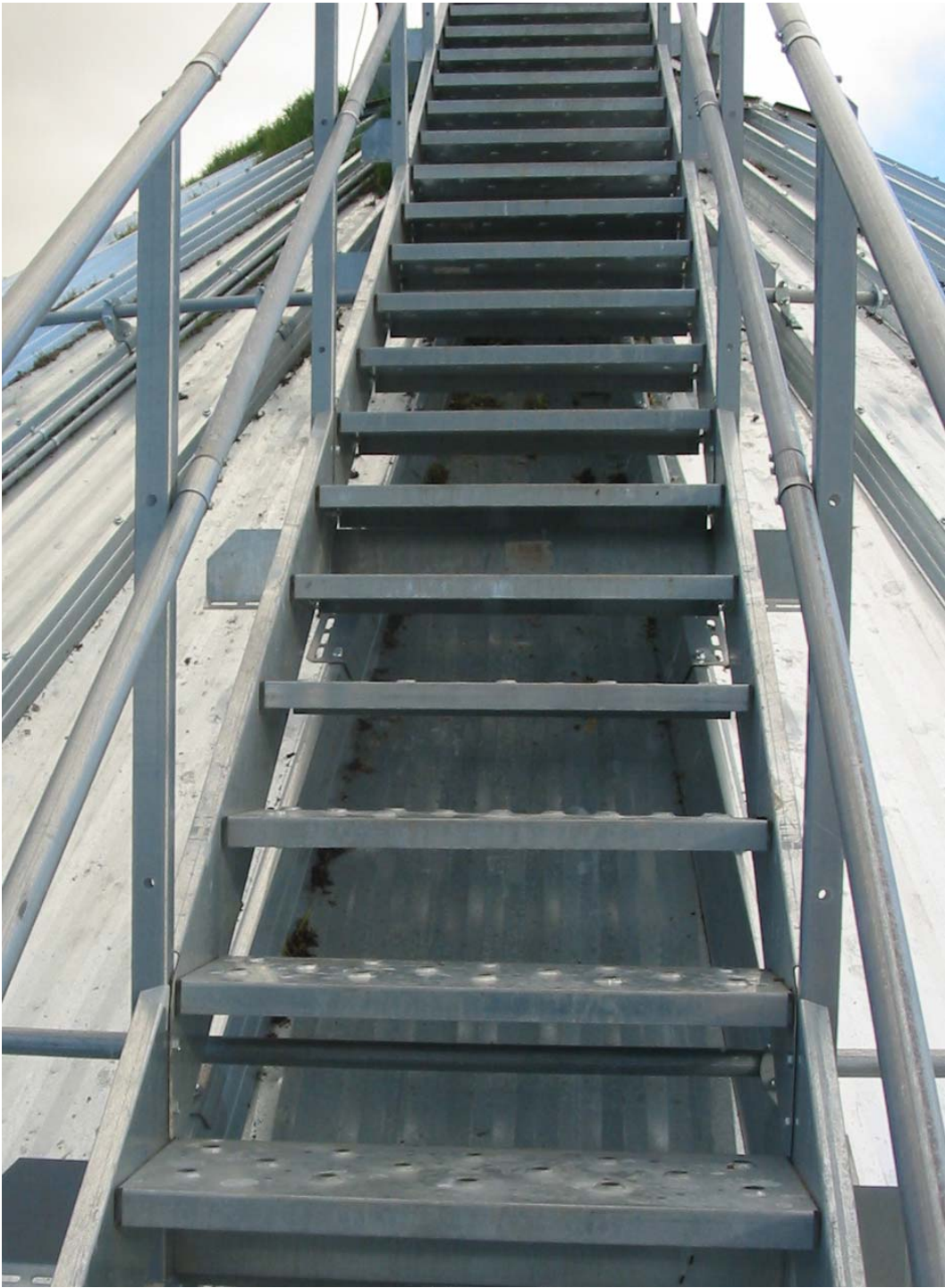
Image 1 – Assembled sections of roof stairs
