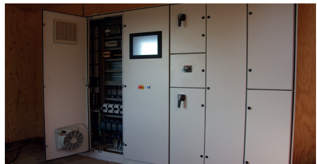
PLC / PC control panel for all sizes of silo installations with more silos and conveyor system.
