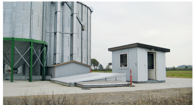
Silo installation with a shed for control panel, distribution board and enough space for a table for crop analysis equipment etc. You can easily inspect the space and intake pit.
