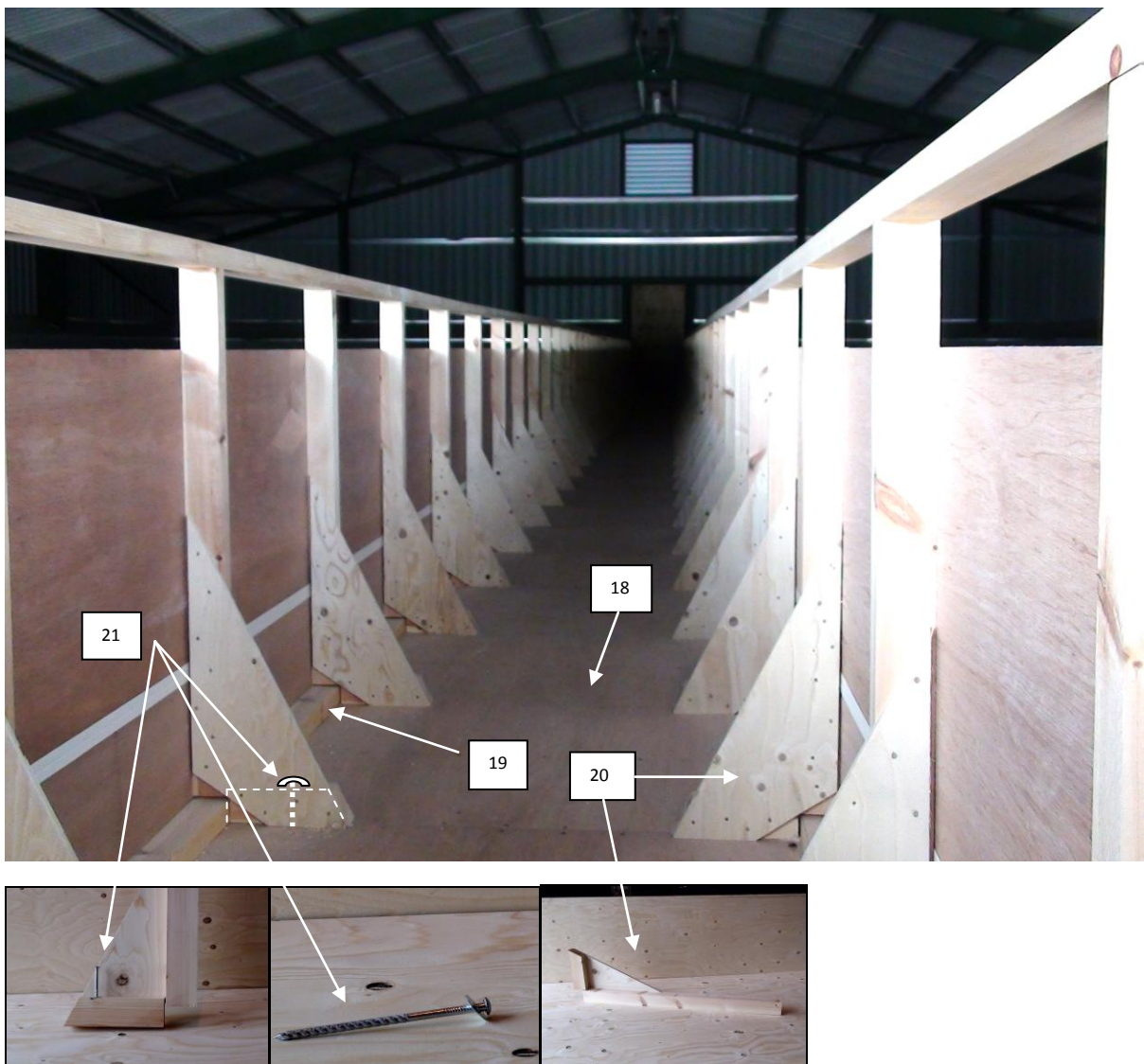
Fig 3 Main Air Duct Walkway
