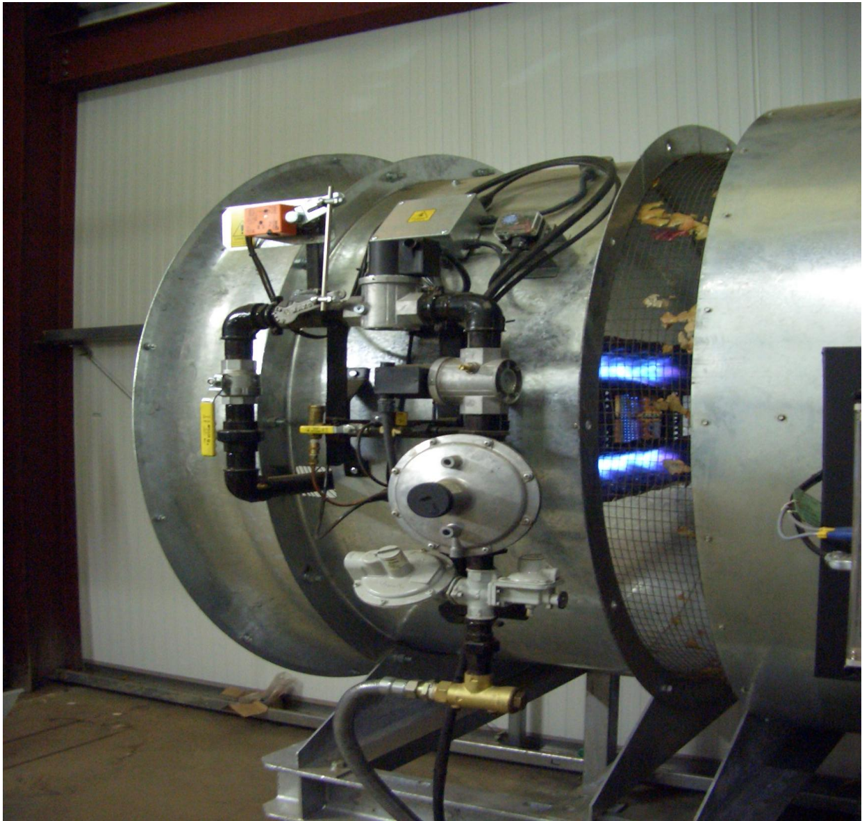
Fig 13 Fully Modulated Gas Burners
